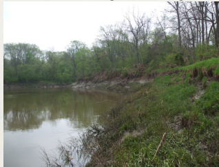
Major slumps have been occurring along the river landing as we lose more soil to the river. (even though we're gaining on the other side of the point bar) Slump scars are now continuous from the mouth of Fleming Creek (seen in the distance) to Mussel Beach (behind camera)
