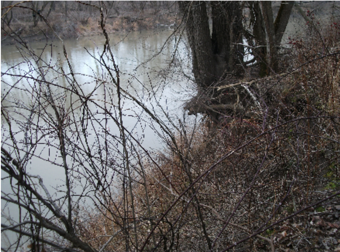
A pair of large Blue Ash trees cling precariously to the river bank with thickened roots, the soil below them being steadily eroded away.
