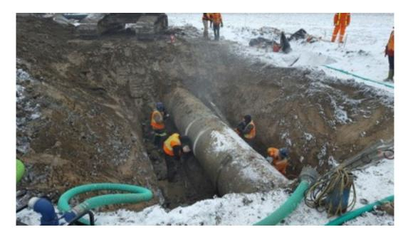
The main water pipeline to London gets a maintenance visit from a work crew. A section of deteriorated pipe was replaced on February 15, causing flow to be shut off for some 18 hours. To find out why our taps didn't run dry, read the following.
